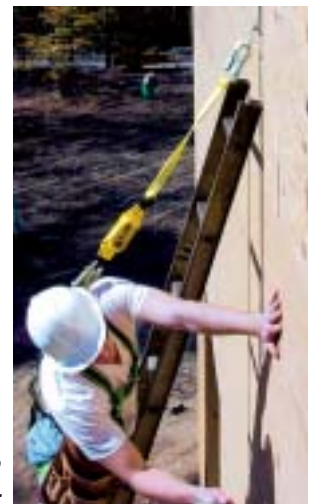
Single D Roof Anchors can also be used for vertical wall applications.
